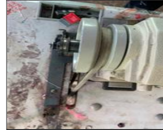
External photo(s) of the production unit(s) NC 7.17 Sewing machine without pulley guard.JPG
